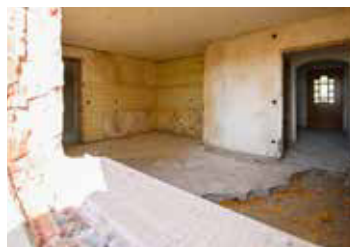
Gutting the old house before demolition
