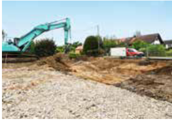
Preparing the building site
