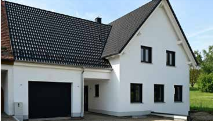
Completion of the new house
