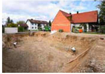
Excavating the construction pit
