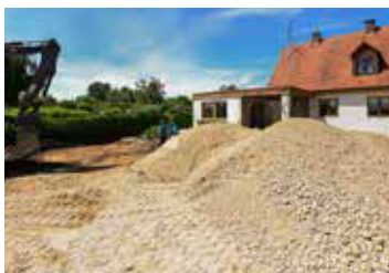
Raising the garden before demolition
