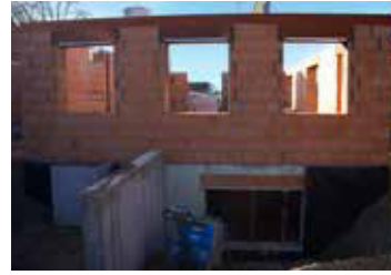
Shell with basement
