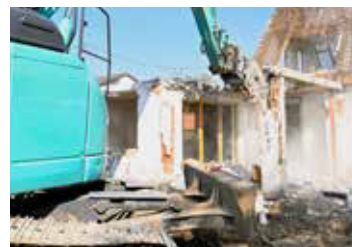
Demolishing the old house
