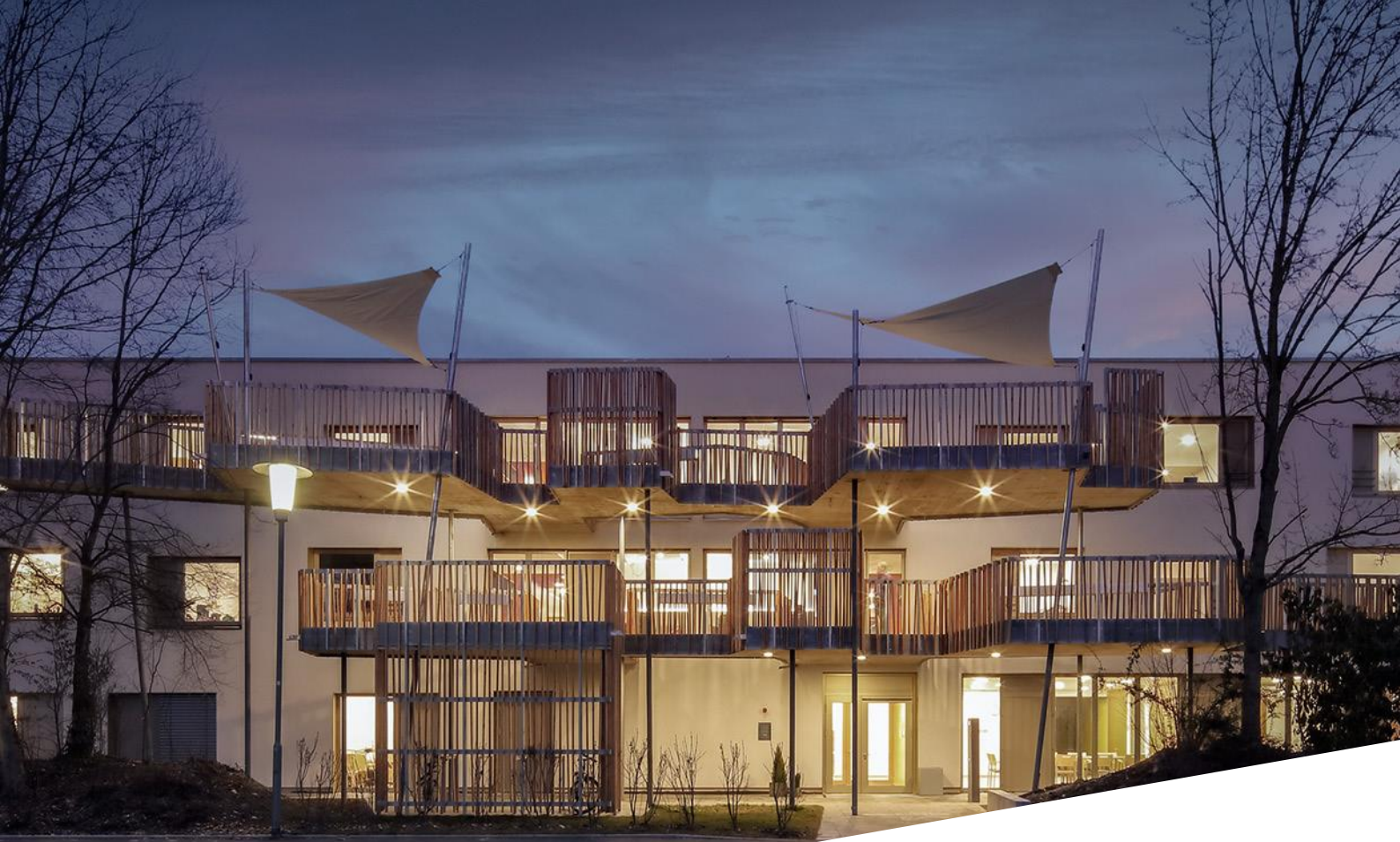
Construction of a new residential home for people with disabilities, Rain a. Lech, Germany Contractor: Stiftung St. Johannes, Marxheim, Germany Planner: UTA Architekten und Stadtplaner GmbH, Stuttgart, Germany Photo: Norman Radon, Ingolstadt, Germany
